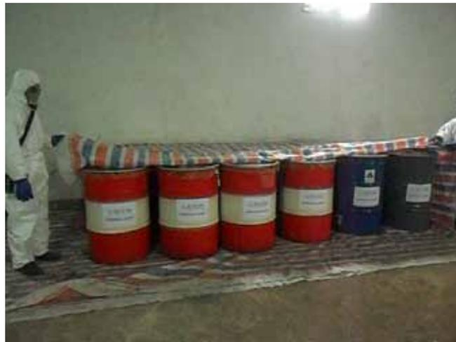
**Fig 3.10 Storage of the asbestos waste collected in the project**
