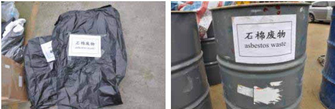
**Fig 3.8 Management requirements of the asbestos waste before transportation**
