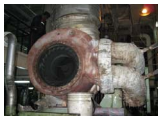
Engine exhaust line (Chrysotile 50%)
