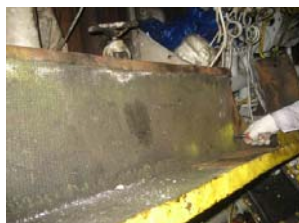
Exhaust cover of generator (Chrysotile 20%)
