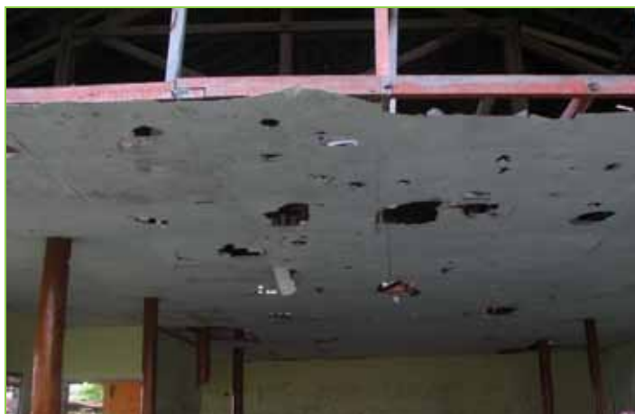
Picture 1. Asbestos Ceiling in Pananjung Sari Hotel
