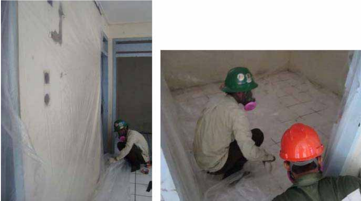
Picture 6. Plastic Barrier Installation
