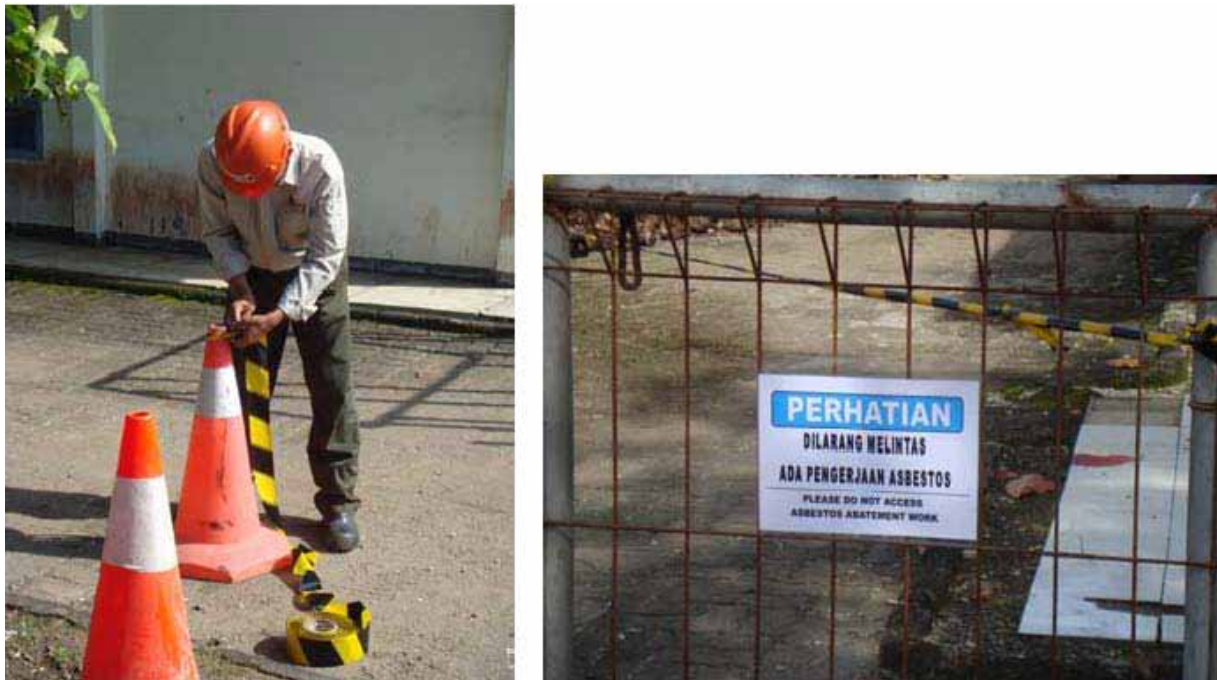
Picture 2. Barricade Line Installation
