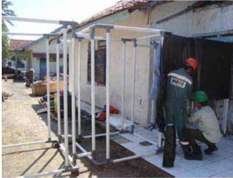
Picture 7. Installation of Decontamination Unit
