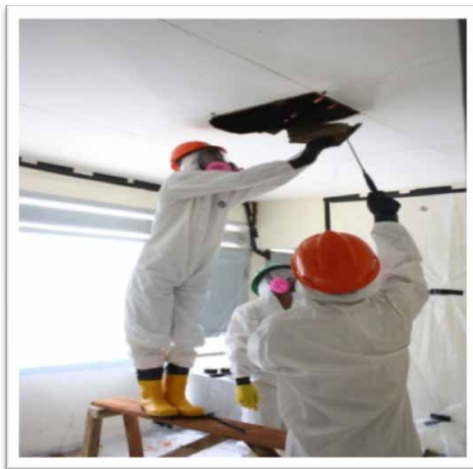
Picture 11. Removing the Asbestos Ceiling
